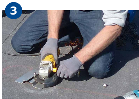
3 Shorten the threaded rod according to the template.
