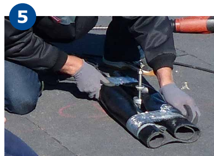
5 Tighten the universal foot directly down onto the threaded rod so there is 100% mechanical connection from the concrete screw to the console system.
