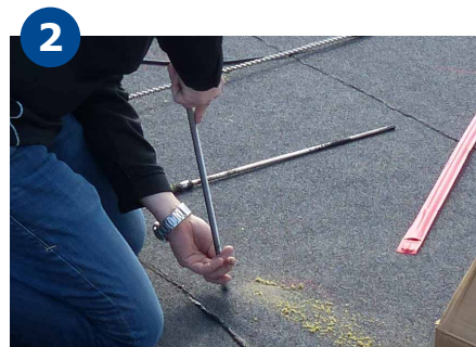
2 12 mm stainless steel threaded rod with pre-mounted concrete screw, screw fully down into the hole.
