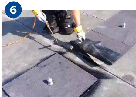
6 Burn the under-felt to seal it according TOR's instructions.
